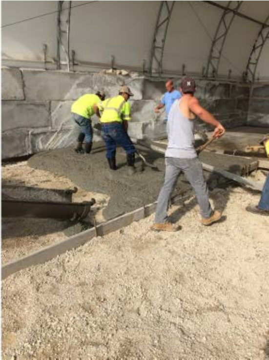
Pouring floor in salt shed
