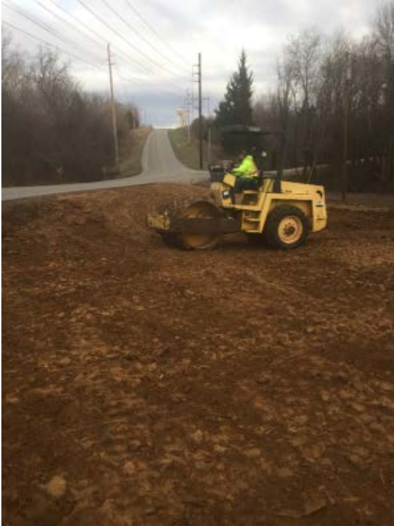
Backfill to straighten South Old Orchard Rd.
