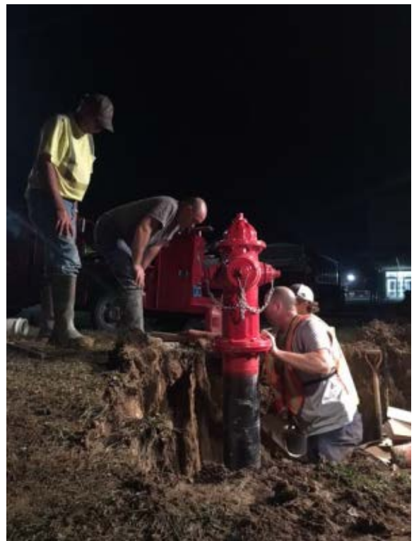
Repairing Fire Hydrant on Kimbel Lane
