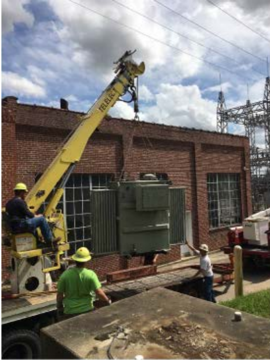
Demolition of old transformer
