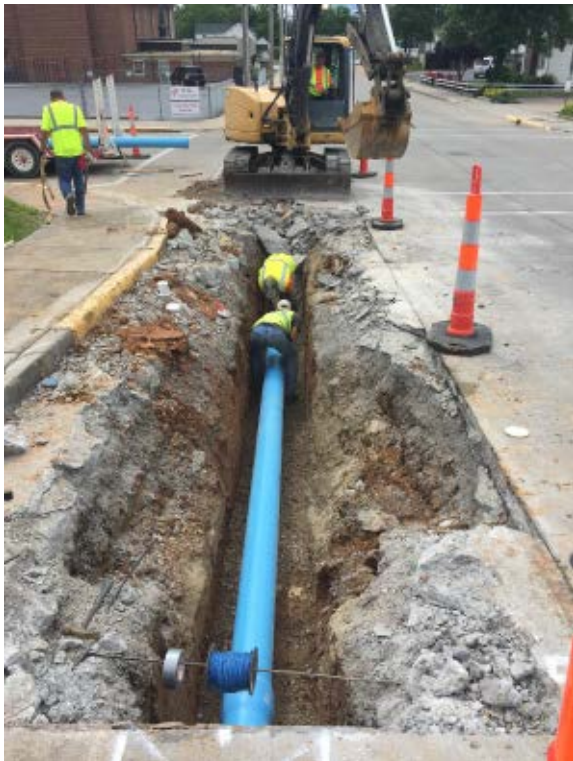
New water main on Adams St. by Nip Kelly Equipment
