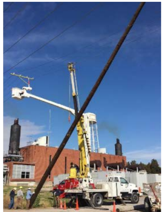
Setting new pole at Power Plant for Transmission and Distribution
